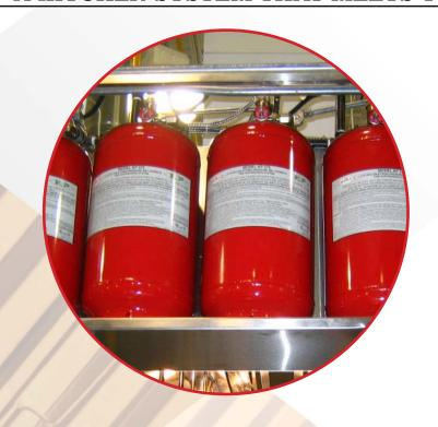
The AMEREX Kitchen Protection (KP) Fire Suppression System has four options for Agent Cylinders, depending on system output needs:
