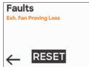
Example of current faults screen, with RESET button
